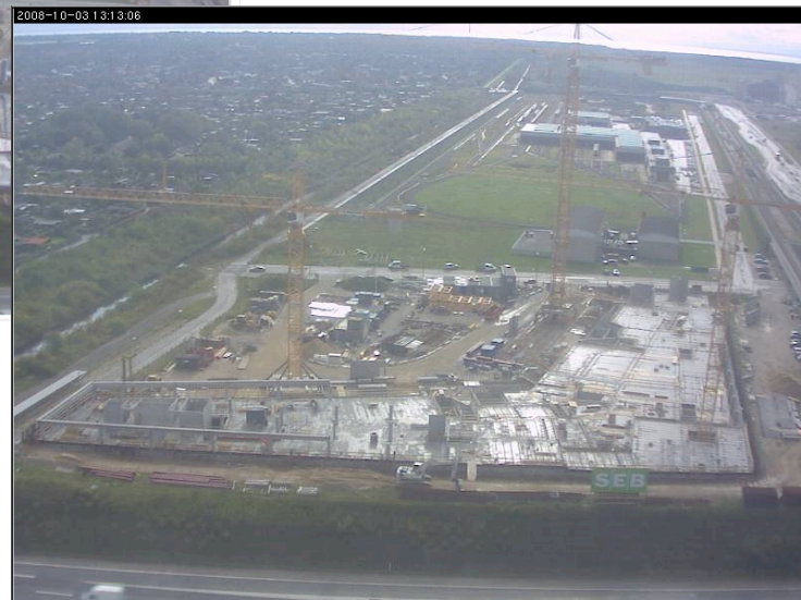
Rambøll new headquarter at Ørestad
